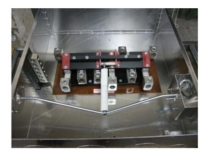
Inspect switch mechanism and note how components look before removing or adjusting components.
